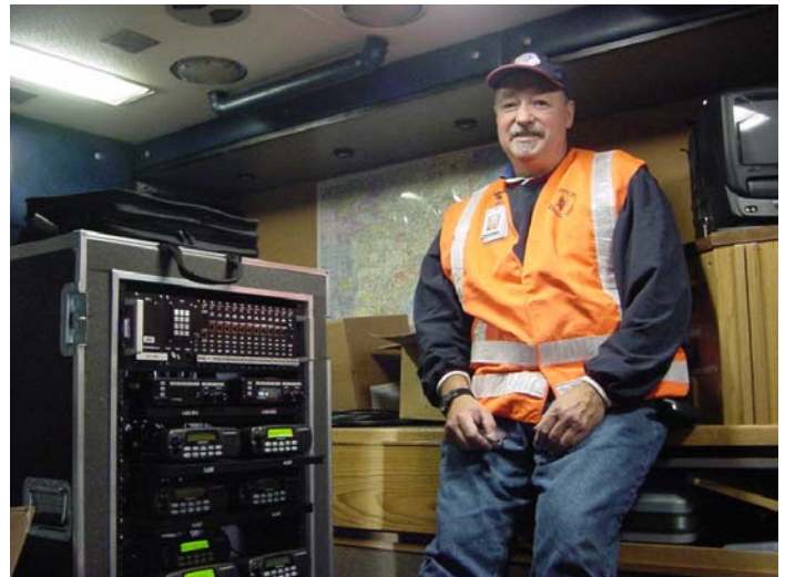
Steve, W8TER, with the ACU-1000 in the ARES truck.
