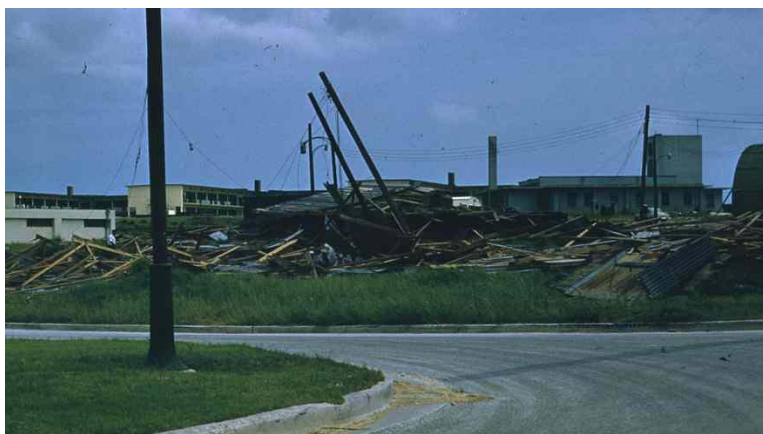
Okinawa typhoon damage.
